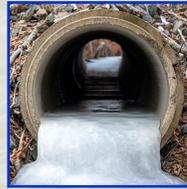
Early in spring we work throughout the County with Steamers (not the drinks) to open up frozen culverts and ensure the water has a place to run. As the summer progresses the water issues turn from freezing issues to beaver issues. For spring, summer and fall the County of St. Paul is in a continuous struggle to keep our culverts and water ways open from damming caused by beavers.
